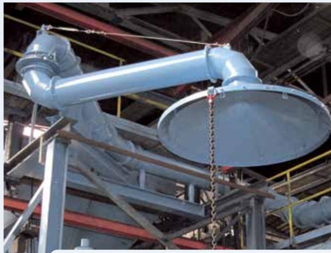
Canopy type Swing Hood for furnace fume extraction system
